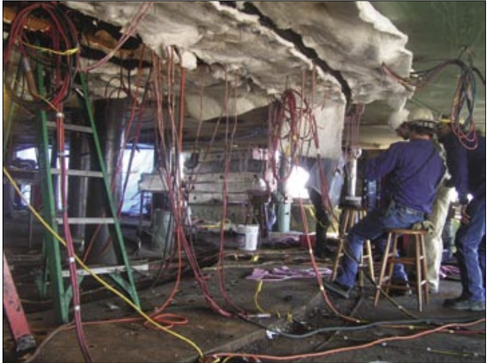
Weld engineers reviewing repair process of dragline base weld.
