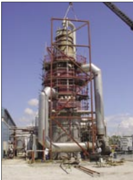
Building the tower framework with bumpers for the Evaporator.
